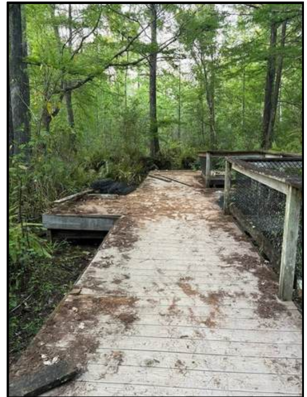
Deconstruction of the old boardwalk is already underway!
